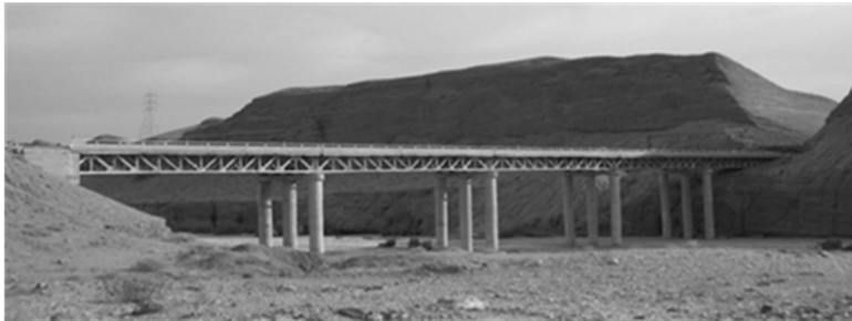
Fig. 1. Aly Dar bridge
